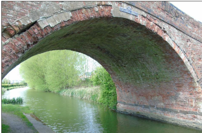
Linear Vistas are important along the canal towpath – Pochins Bridge looking towards Pochins Bridge housing.
