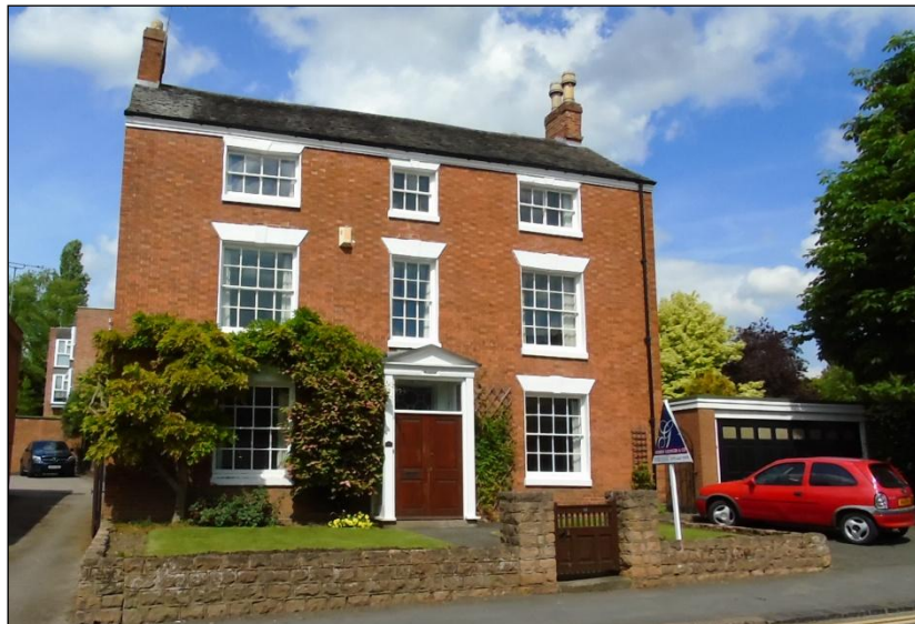
Three storey house on London Road, Oadby showing traditional features.
