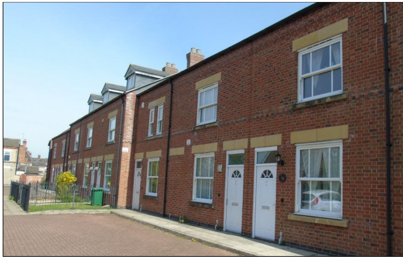
New housing association development on Countesthorpe Road, South Wigston demonstrates effective and careful reflection of its built environment context.
