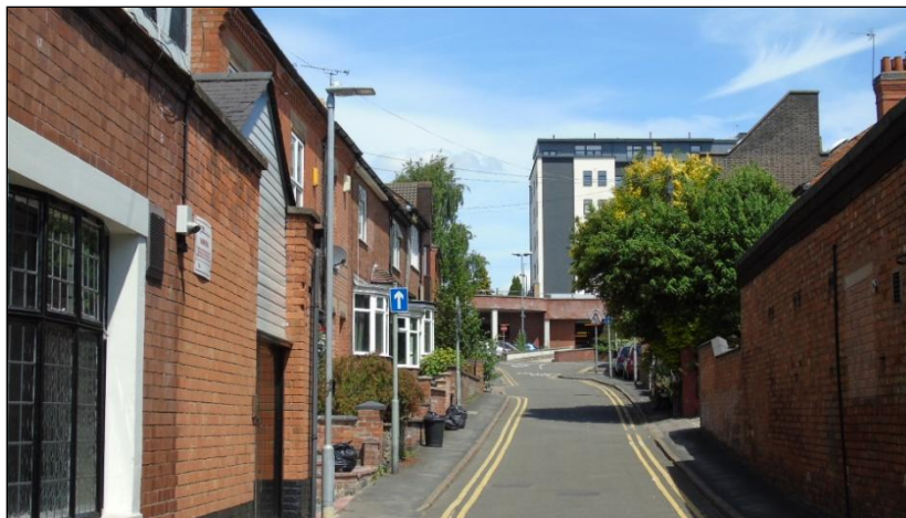
The view up Albion Street gives an idea of the original character of the settlement and shows the impact of inappropriate development.
