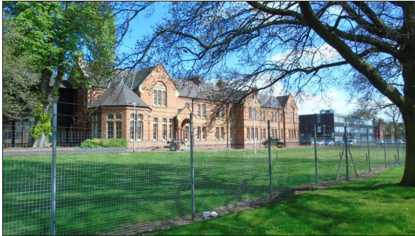
The 'Institutional Character' of the area is clearly apparent from the Territorial Army Headquarters.
