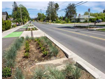
Low-level rainwater garden
