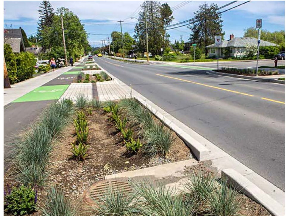
Figure 7.6 – Example of a rainwater garden in Vancouver, Canada
