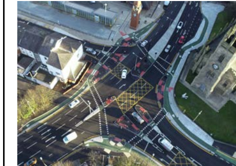
FIG 3 - EXAMPLE OF "CYCLOPS" JUNCTION SOURCE: https://beeactive.tfgm.com/schemes/bolton/newport-street-cyclops-junction-bolton/ ACCESSED ON 14/09/22
