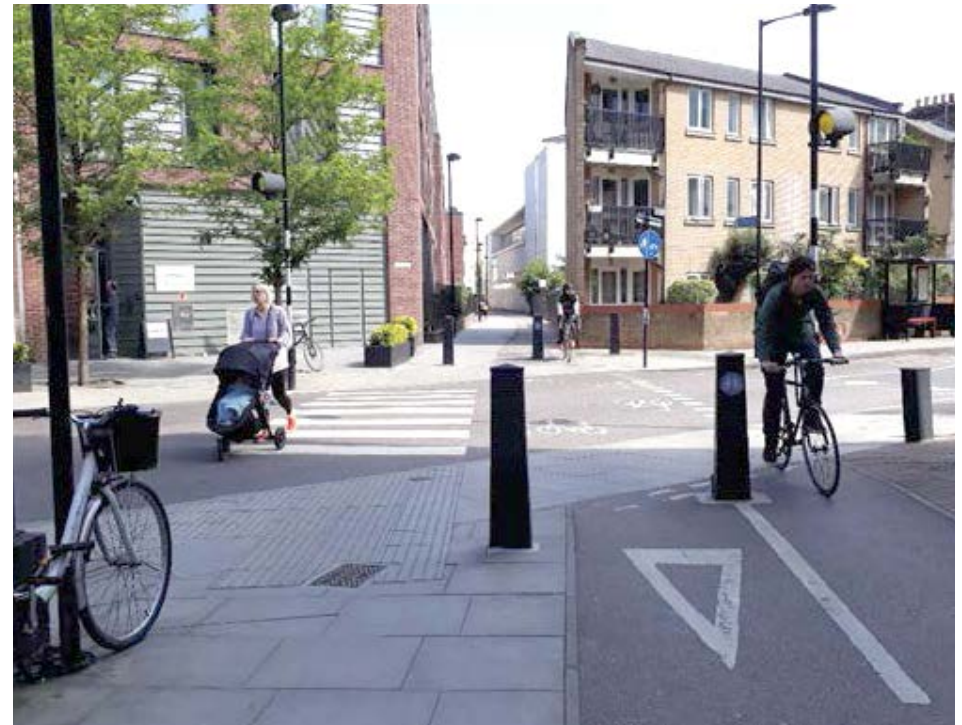
Figure 7.8 – Example of a raised crossing in Hackney
